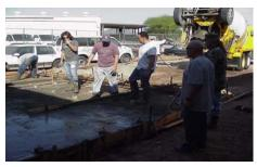
A Building Construction class poured concrete as part of a lab project that will be used in the Industrial Technology Division. Students got handson experience in learning methods of pouring and finishing concrete.
