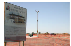
North Parking Lot Construction
